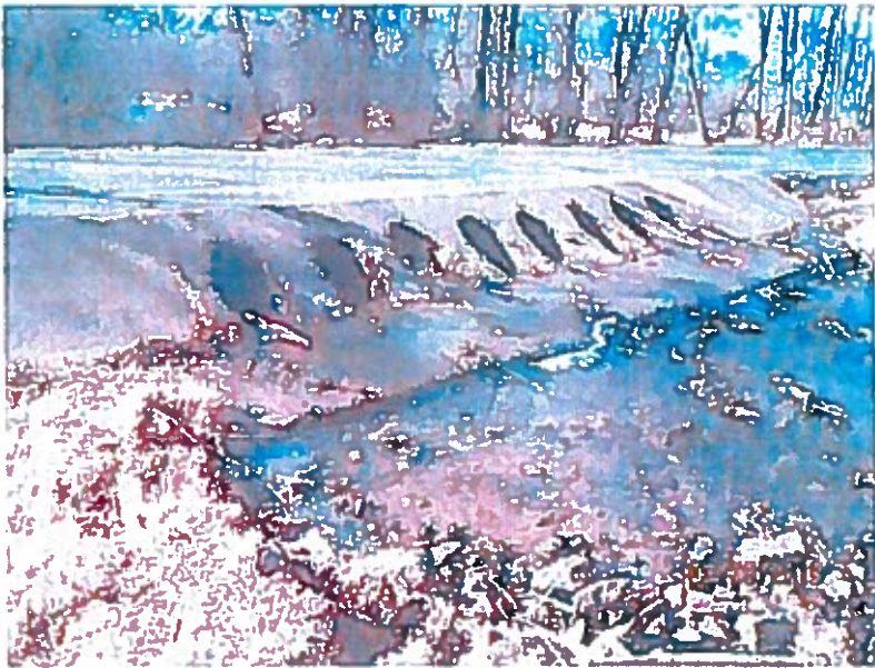
General condition of pipe outlets and endwall.
